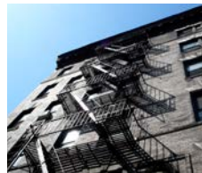
Building, 2007 © Dan Hill
