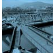
PEDRO ARRUPPE BRIDGE
