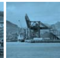
PORT (1ST PHASE)
