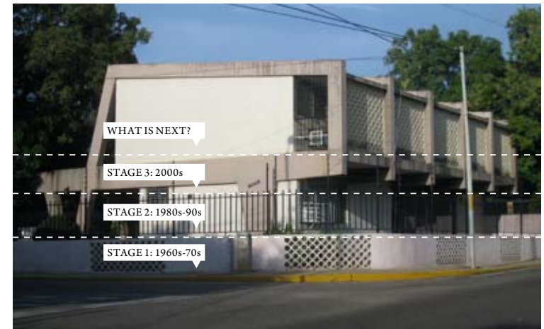
Fence stages in a residential building
